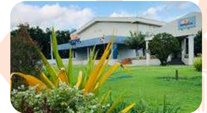
Sunquick RTD Factory, Horana Provision Total Plumbing Services
