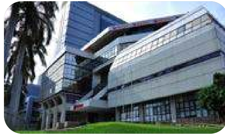
National Development Bank VRV System
