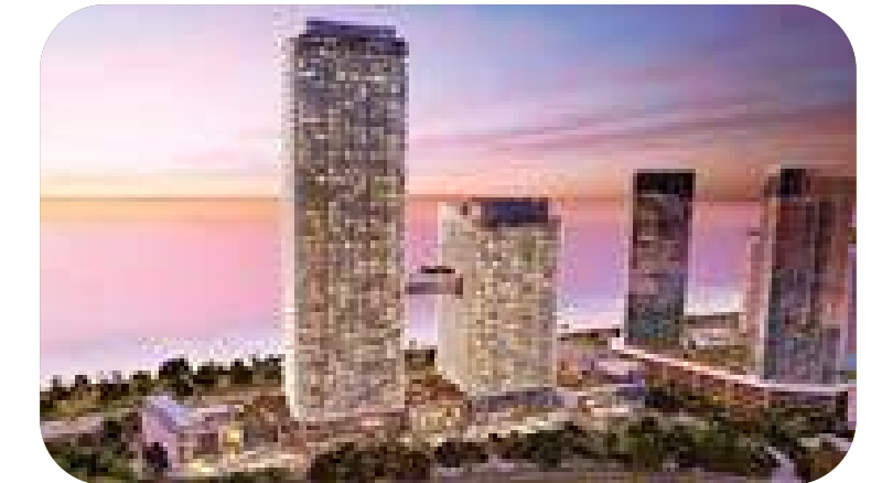
ITC One Colombo Fire Protection system Installation - Hotel Scope
