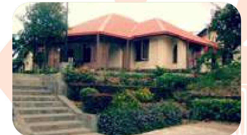
Hillwood College - Kandy Auditorium Sounds, PA and Stage Lighting System
