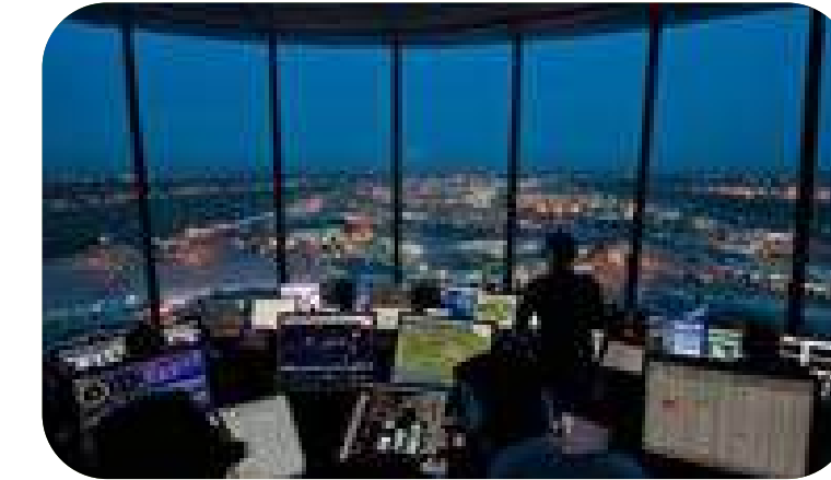
AASL - Air Traffic Control CAPACITY: 320 KVA
