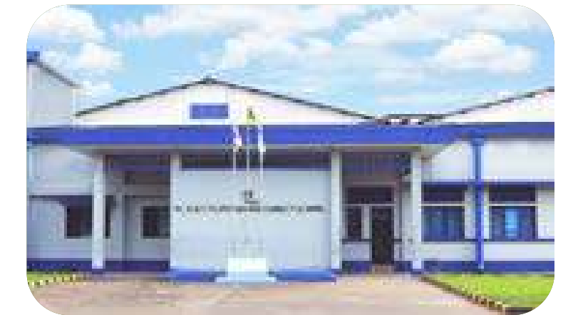
South Asia Textiles Ltd Central AC Chiller System
