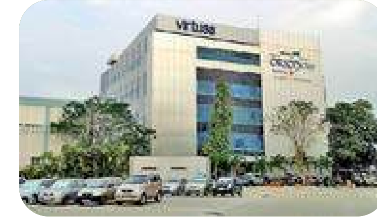
Virtusa Corporation CAPACITY: 840 KVA
