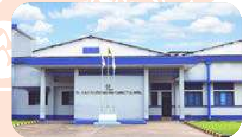
South Asia Textiles Central AC Chiller System
