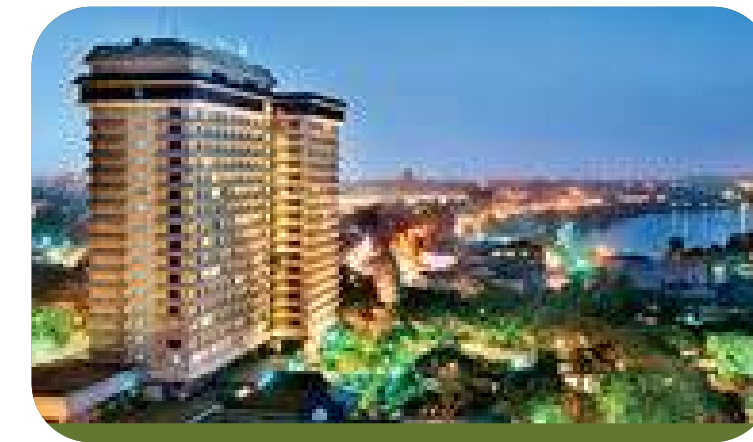
Hilton Colombo Central AC Chiller System
