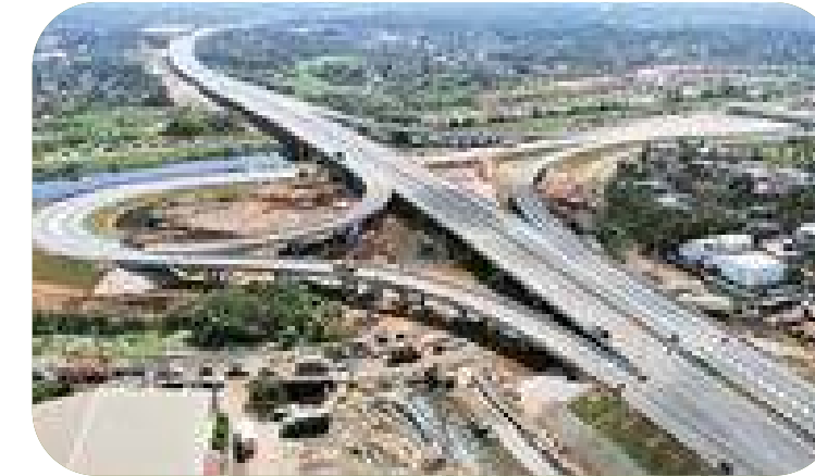
The Southern Expressway IPCCTV System with central monitoring station including the Network
