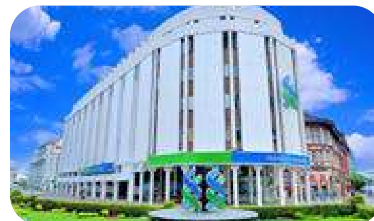
Standard Chartered Bank (for CBRE South Asias (Pvt.) Ltd.) Electrical Services | Mechanical Services Civil and Plumbing Services Building Management Services
