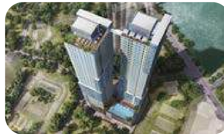
Capitol TwinPeaks Total Electrical Services
