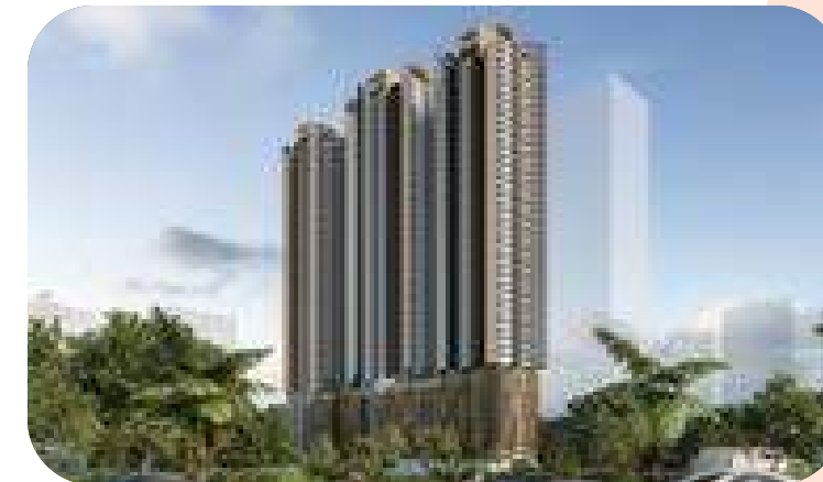
Trizen Apartment Tower 02- total plumbing system Installation
