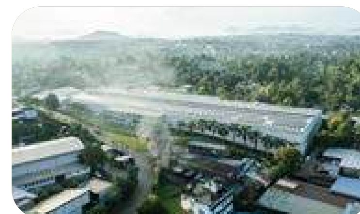
Lanka Tiles PLC CAPACITY: 550 KVA
