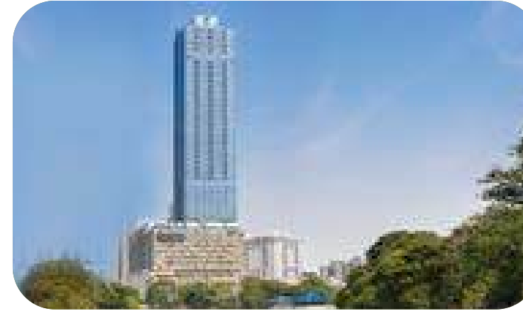
Colombo City Centre Total Electrical Services
