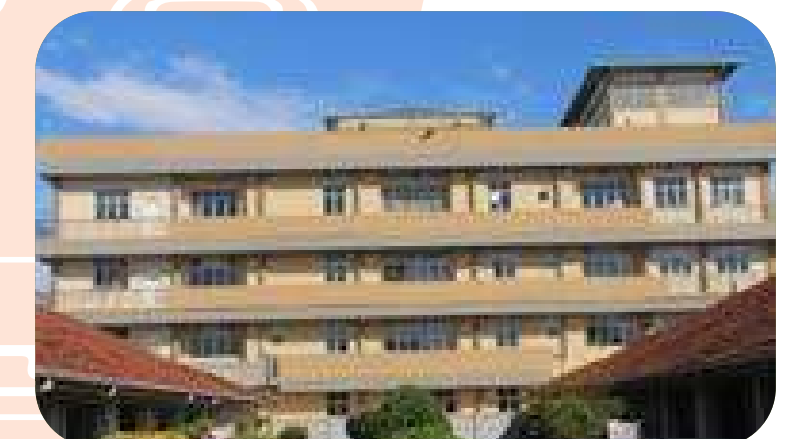
Castle Street Hospital Electrical services
