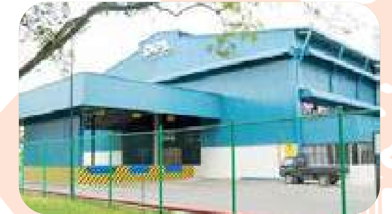
DPL Premier Gloves Pvt Ltd Provision Supply of Booster, Submersible and Fire Pumps
