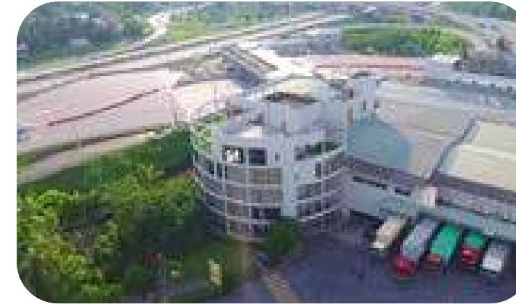
Ceylon Biscuit Limited CAPACITY: 1600 KVA
