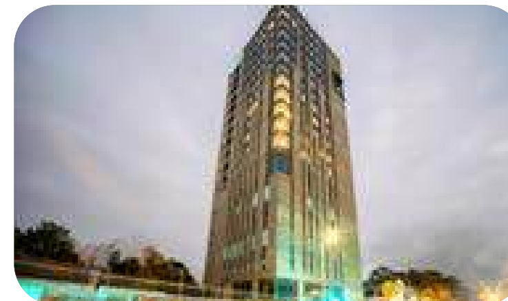
AOD Colombo Innovation Tower Total Plumbing Services
