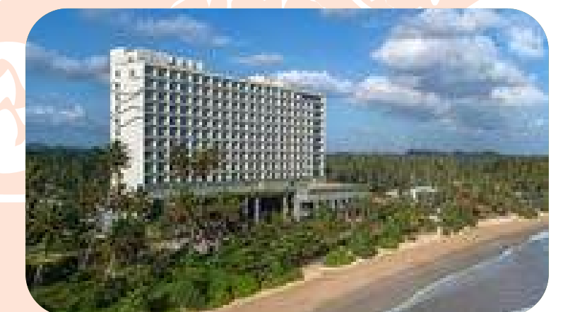
Marriot Resort & Spa Designing of Electrical Systems Winner of CIDA Award for installation excellence
