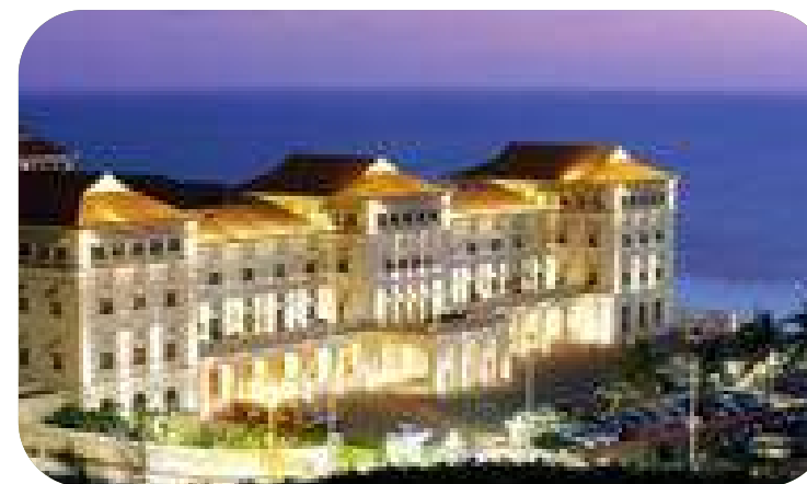
Galle Face Hotels Total Eaelectrical Services
