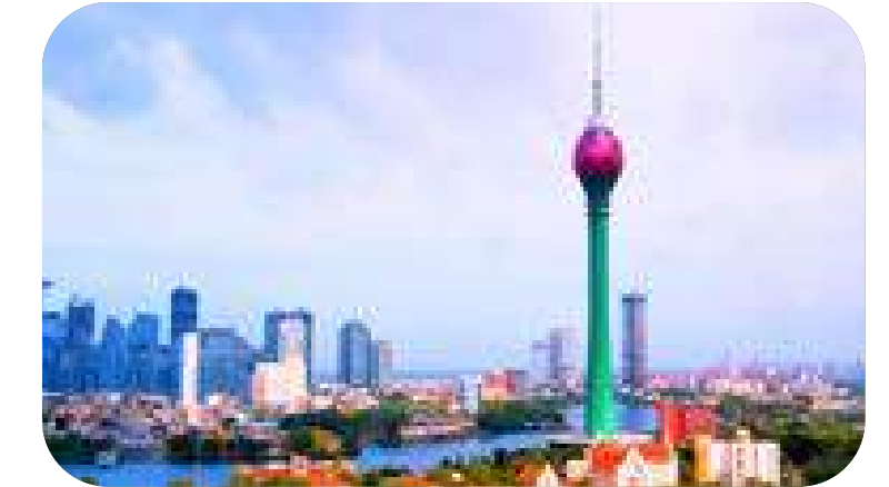
Lotus Tower Integrated CCTV system with over two hundred cameras
