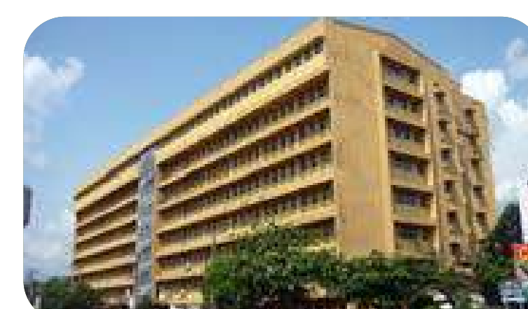
District General Hospital, Gampaha Central AC Chiller System
