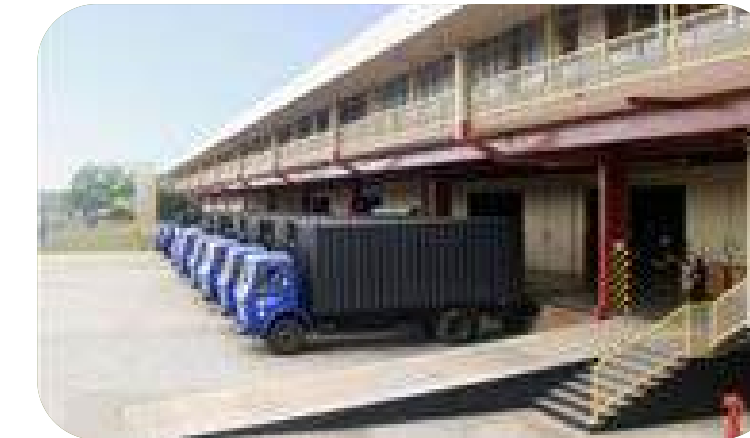
Logiwiz Warehouse Kotugoda Phase 01 and Phase 02- Total Fire Protection and detection solution
