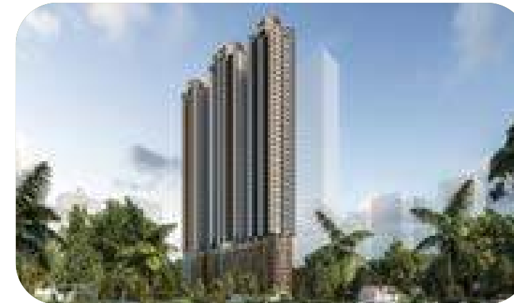
Trizen Apartment Total Fire Protection and detection Services
