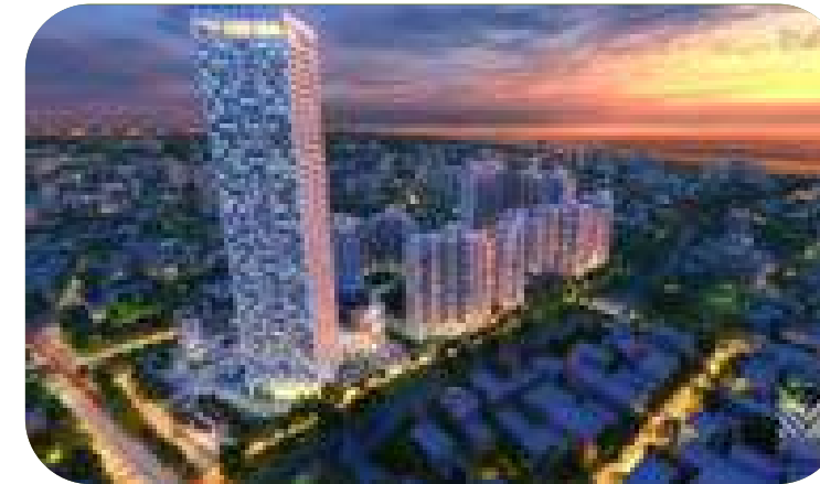
HSBC Mireka Tower Fire Protection system, Suppression system and Aspiration system
