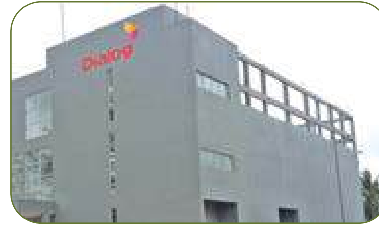
Dialog Data Centre Central AC Chiller System
