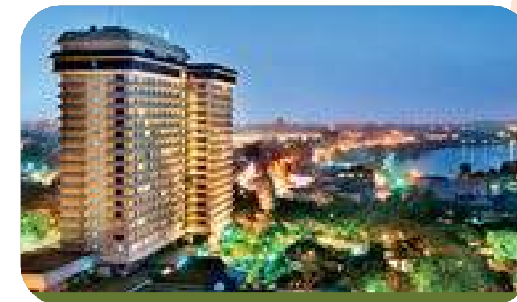
The Hilton, Colombo PA and Pipe Music System for the premises IPCCTV System, Data Network System Voice Telephony System
