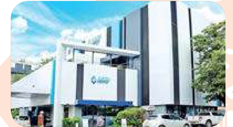
Asiri Hospital PLC CAPACITY: 280 KVA
