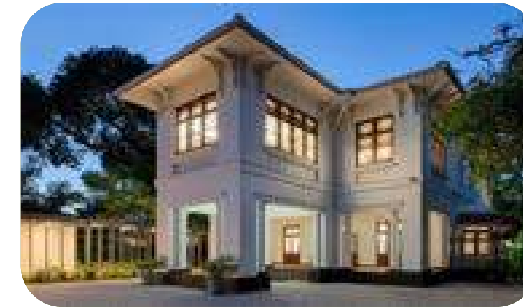
The Embassy of Switzerland in Sri Lanka Integrated Security System comprising of IPCCTV system
